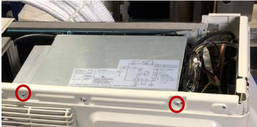
Lift electrical box out carefully disconnecting wire harnesses along the way.
